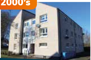
External Wall Insulation, Denny
